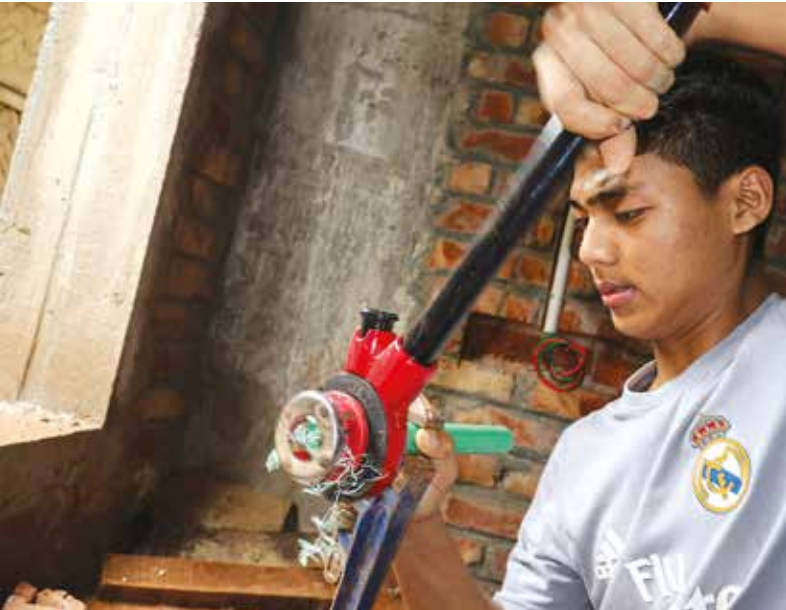
Youth Skill Development - Plumbing & Pipe Fitting, Newton Chakma, Jurachari, Rangamati Photo : Anindeta Chowdhury
